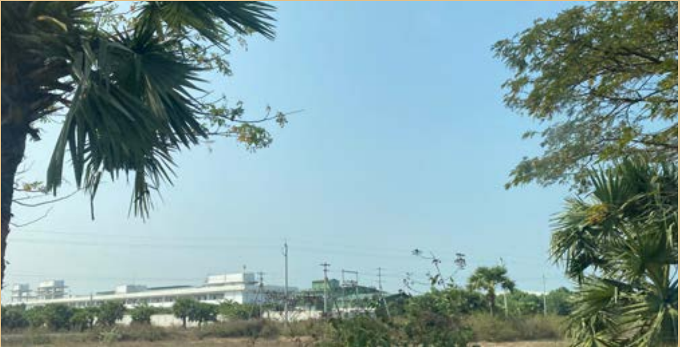
A large shrimp processing facility (Andhra Pradesh, 2024)
