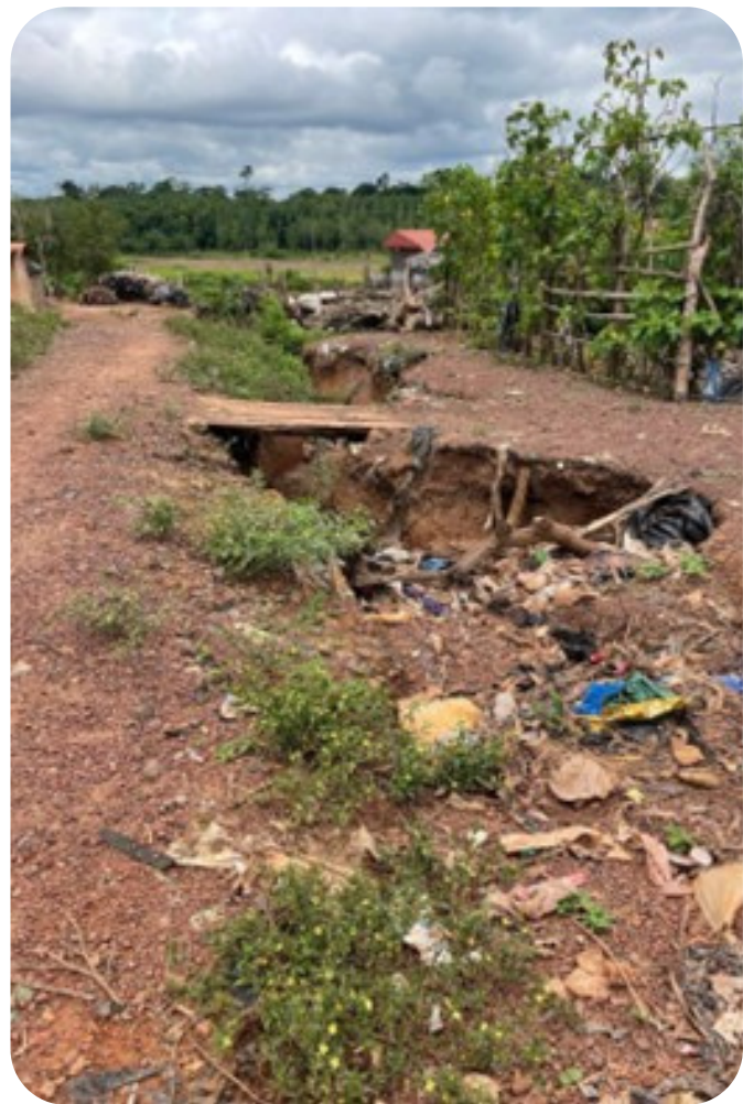
A road, rendered impassable by rain and erosion, leading out of a village in Côte d'Ivoire (September 2022)
